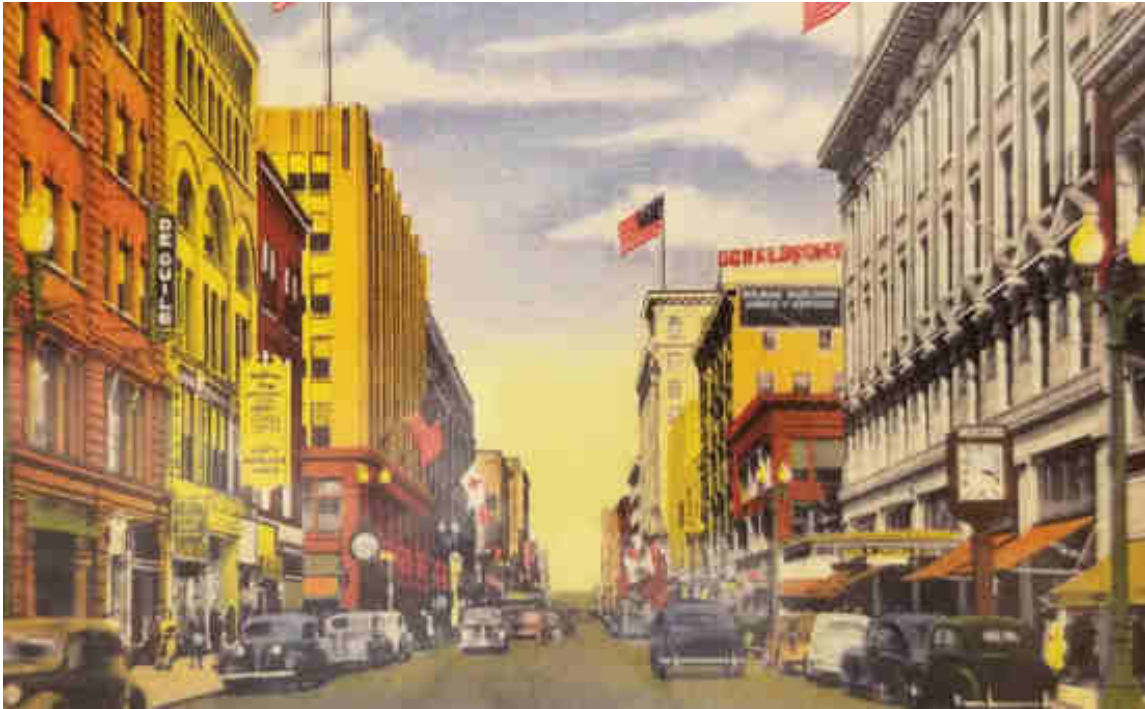
Nicollet Ave. looking north, Minneapolis, MN.
